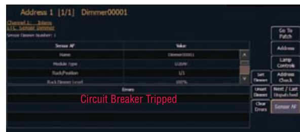
Figure 3: EOS ACN feedback for dimmer circuit breaker trip error
